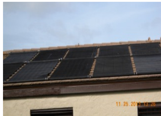
SOLAR HEATING PANELS
