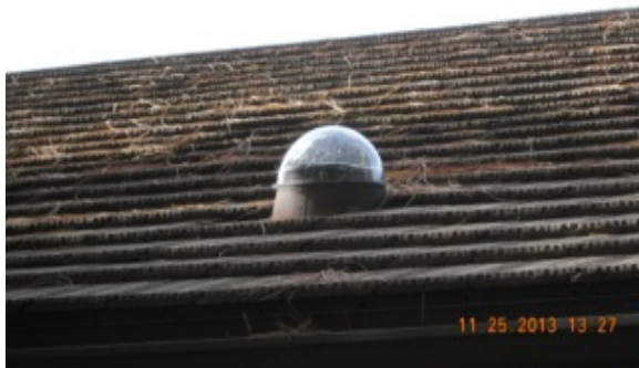
SOLAR TUBE SKYLIGHT
